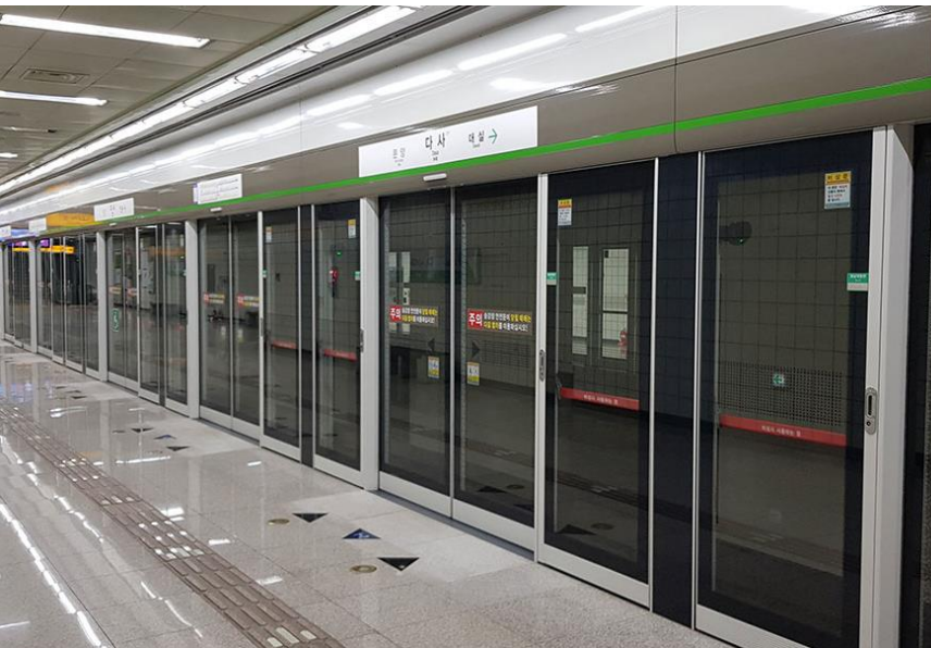
Platform Screen Door
